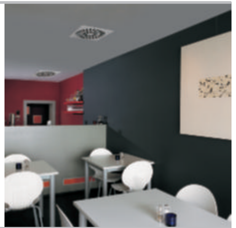
Concealed ceiling unit >
