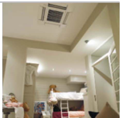
4-way blow ceiling mounted cassette > (600x600)
