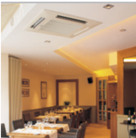
< 4-way blow ceiling mounted cassette (950x950)
