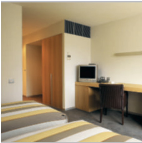
< Concealed ceiling unit
